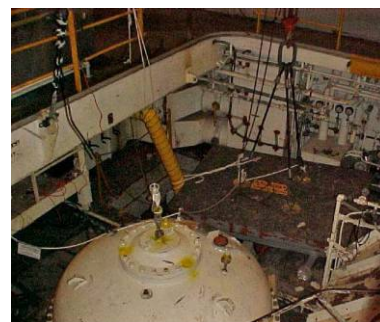
The spent fuel tank of the Sturgis , used as a garbage bin for a radioactive waste issued from the cleaning of the ship © US Army
