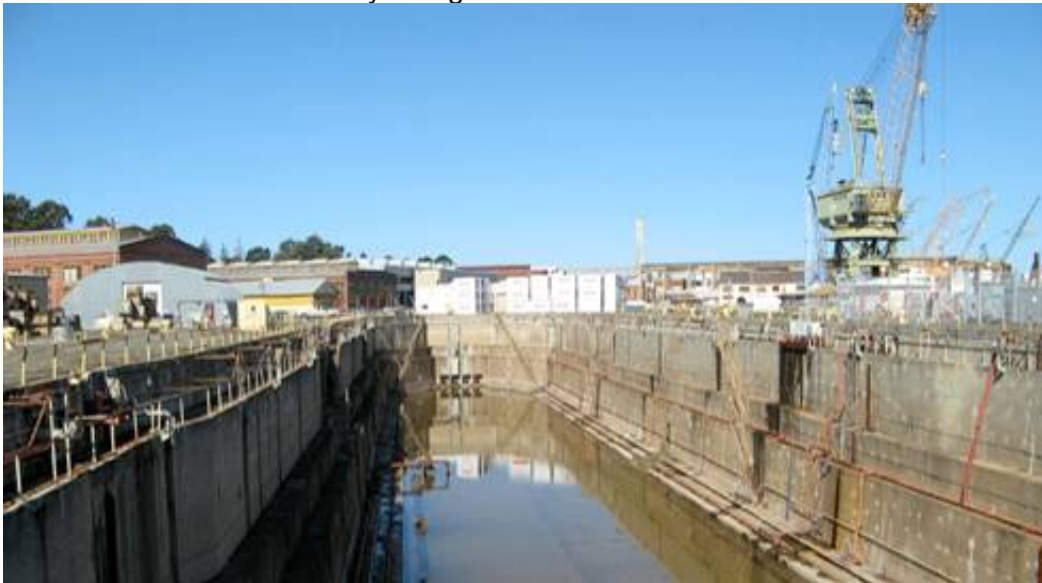
One of the dry docks at the former Mare Island naval base © San Francisco Bay Crossings
