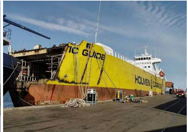
February 2012, ship-breaking in Grenaa (Denmark) © Bendt Nielsen
