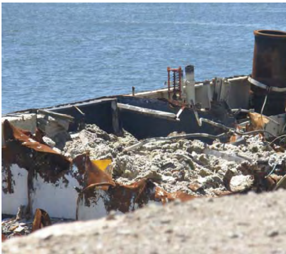
Waste inside the F 484
