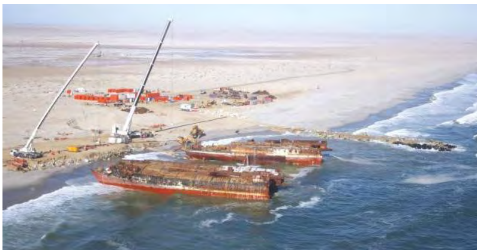
April 2013, to facilitate demolition the Chamarel was cut in two ©Allgemeine Zeitung-Namibia
