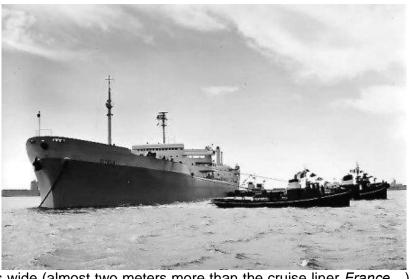
The ship is 259 meters long, 35,6 meters wide (almost two meters more than the cruise liner *France...*), 18,40 meters deep and her draught can reach 13,87 meters. She is propelled by two turbines totaling 24,000 horsepower at the speed of 16,5 knots.
