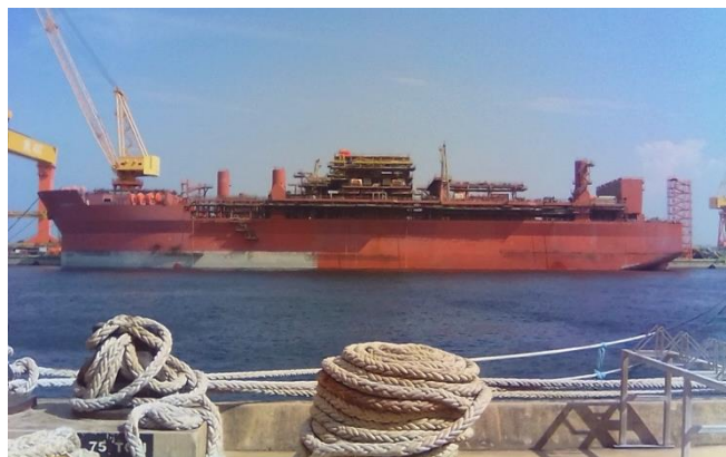
Camburi , July 2017, construction has stopped. © Robert Radziszewski
